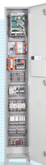
STEP® Elevator Serial Integrated Controller
